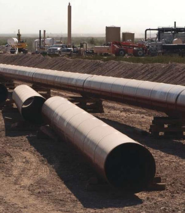
Vaquero is laying 100 miles of trunk pipelines to serve associated gathering lines. Portions of the new system entered service in late 2015.
